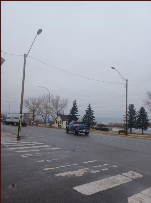
Improved HWY2N intersection lighting for pedestrians.
