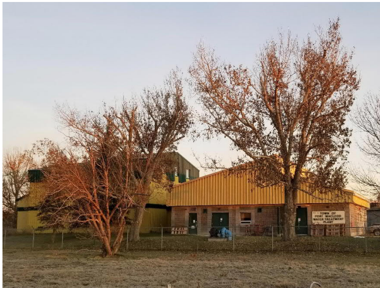
Figure 3.4 – Fort Macleod Water Treatment Plant
