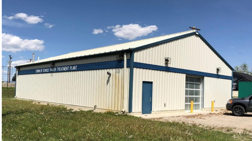
Figure 3.2 – Stavely Water Treatment Plant
