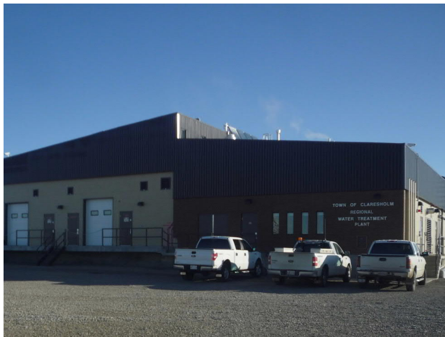
Figure 3.3 – Claresholm Water Treatment Plant
