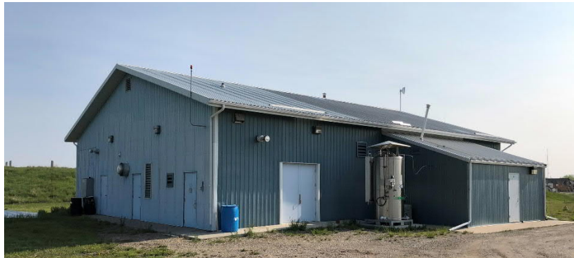
Figure 3.1 – Nanton Water Treatment Plant
